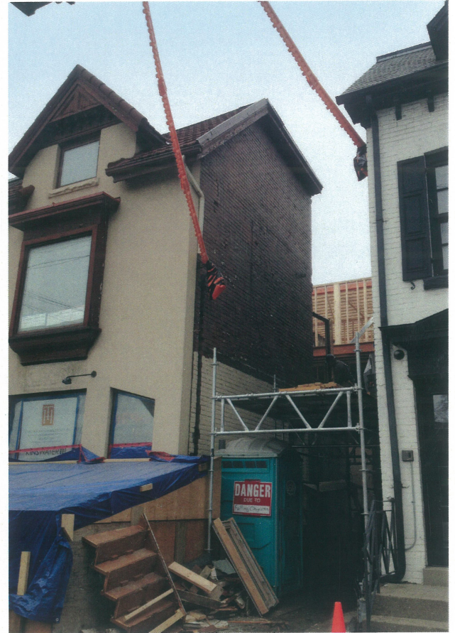
With limited access manpower was the name of the game. Wheelbarrows moved concrete and soil for underpinning. Red iron was moved and placed by hand.
